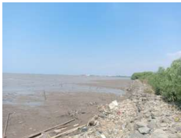
Figure 8. Condition of Kesenden Beach
