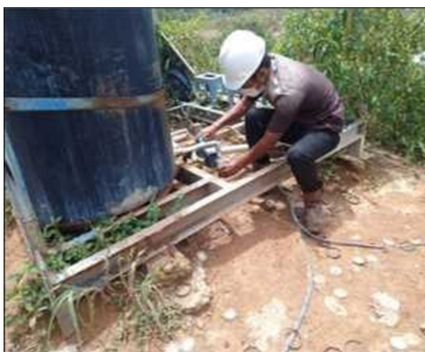
Figure 10. Chemical Organic Coagulant Discharge Measurement
