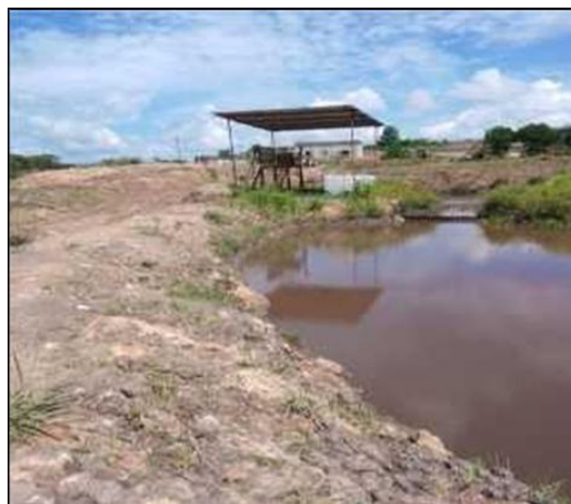
Figure 8. Chemical Organic Coagulant Mixing and Mixing Place on Outlet Channels
