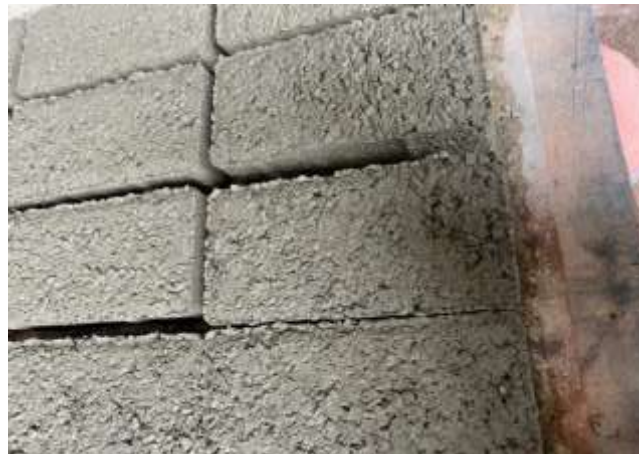
Figure 3 Paving Block Variation 15%
