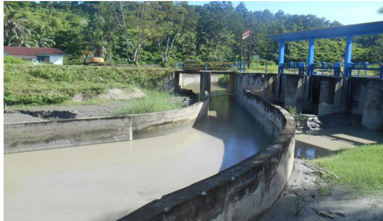
Figure 1 Mud bags that do not function normally (Source: doc, 2024)
