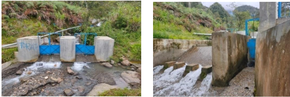
(c) Intake Eksisting
