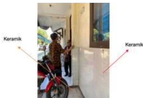
Figure 8. Dormitory Building Materials Wyata Guna Center (B)
