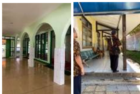
Figure 9. Building Column Repetition Wyatt Guna Center
