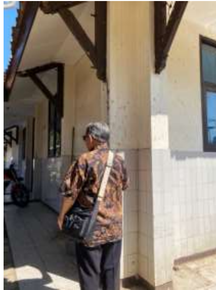
Figure 12. Column Structure Wyata Guna Center Dormitory (B)
