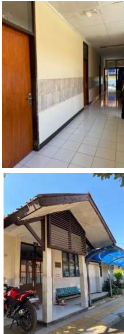
Figure 16 Interior and Exterior Colors of the Wyata Guna Center Dormitory (B)
